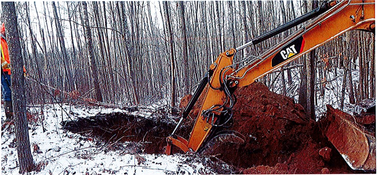
Photo 2 - Test Pit 1 excavation on ridge.
